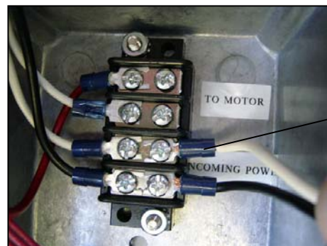
Connect Neutral lead into corresponding connection
