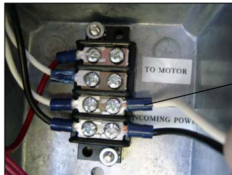
Connect Neutral lead into corresponding connection
