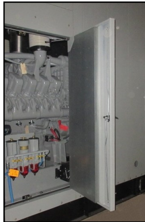
Left: Acoustic foam, visible on inside door panel, reduces noise output on Sound-Attenuated Enclosures. Right: Motorized louvers, visible before addition of intake hood.
