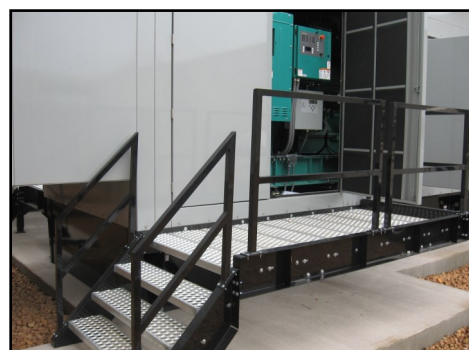
Walkway and Platform installed on Enclosure Package.
